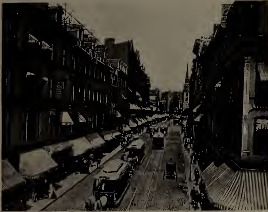
WASHINGTON STREET, north, from Summer. The principal retail thoroughfare.
